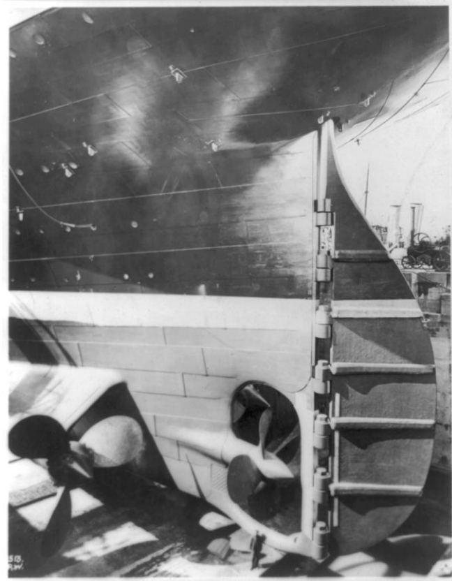
Titanic's rudder - used to steer the boat. Tiny compared to the rest of the ship! Did this affect the steering? 1911
